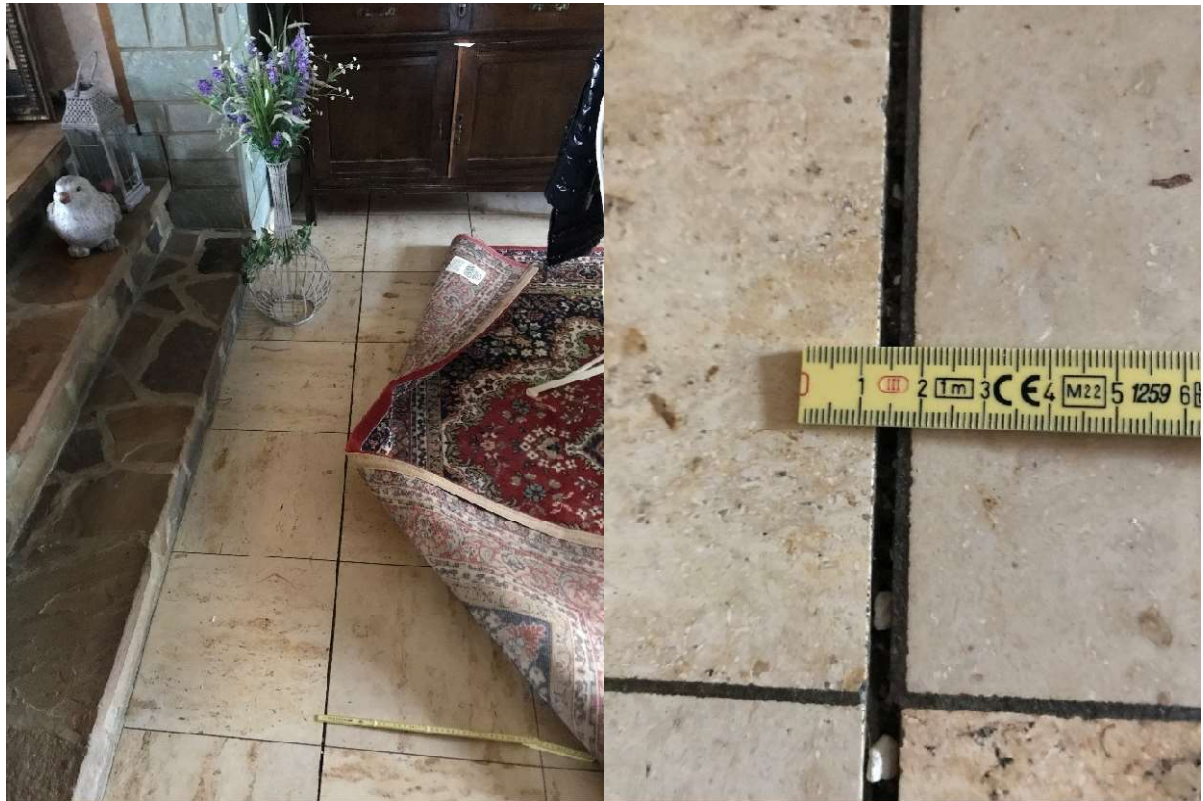
Figure 16 : Fissure D.8
