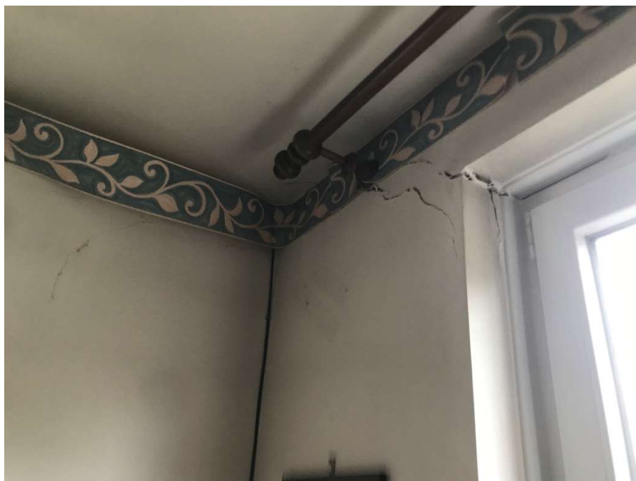
Figure 9 : Fissures D.1
