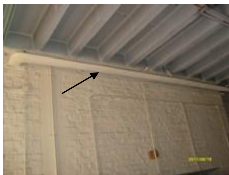
Photo 32 (calorifuge – local bricolage)
