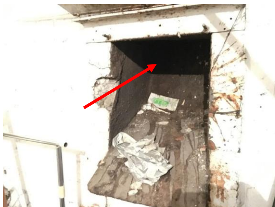
Bron 14 : asbestkokers (asbestcement)
